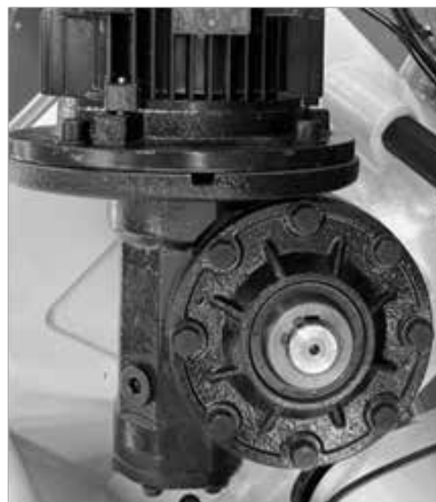
Fig.18 Gear Box Cleaning
